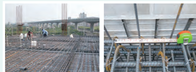
10 樑板鋼筋綁紮
